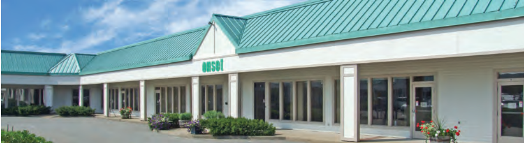
Onset headquarters, Cape Cod, MA
