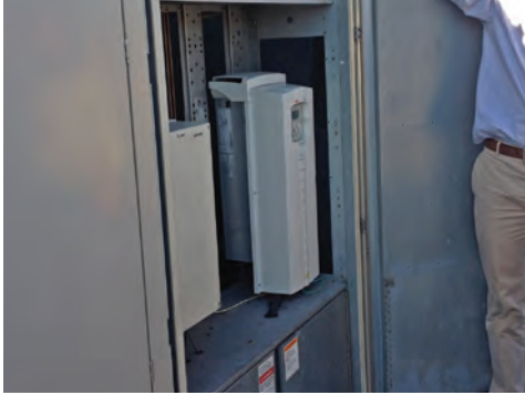
Variable frequency, or speed drives.
